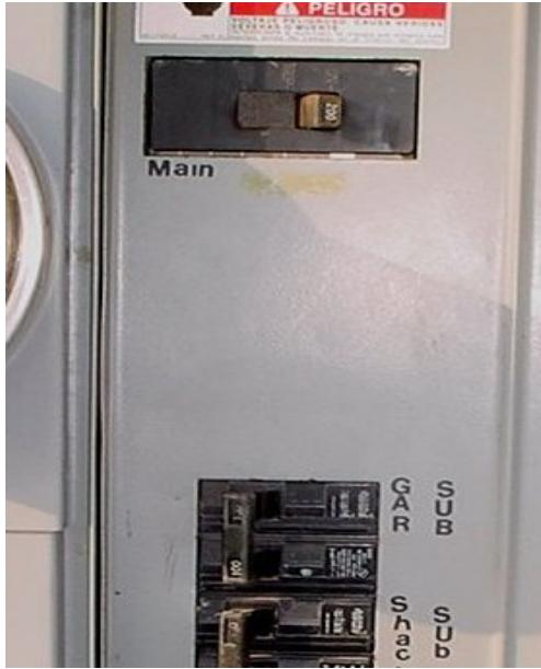
9) With the panel cover firmly in place test the *InterLock kit* to make sure that it transfers easily between positions. **BOTH BREAKERS SHOULD NOT BE ABLE TO BE IN THE “ON” POSITION AT THE SAME TIME.** Even with moderate pressure you should not be able to engage both breakers at once.
