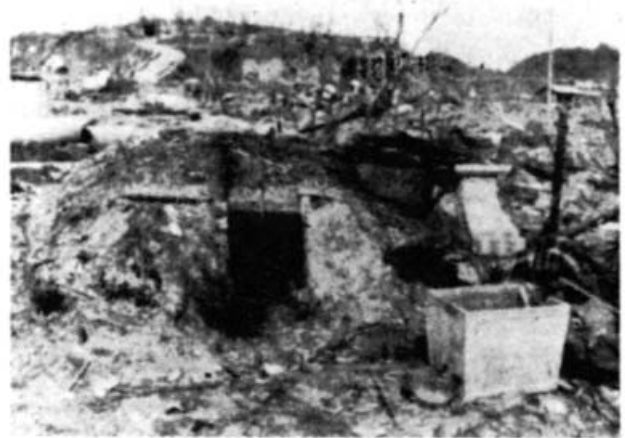
Fig. 1.5. Undamaged earth-covered family shelter in Nagasaki.
