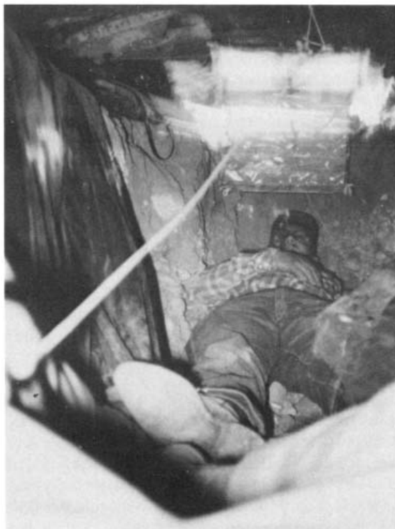
Fig. 6.3. Pulling a Small, Stick-Frame KAP to Keep Temperatures Endurable for Occupants of a Car-Over-Trench Shelter in Warm Weather. Enough air also can be supplied with a small Directional Fan, although more laboriously.
