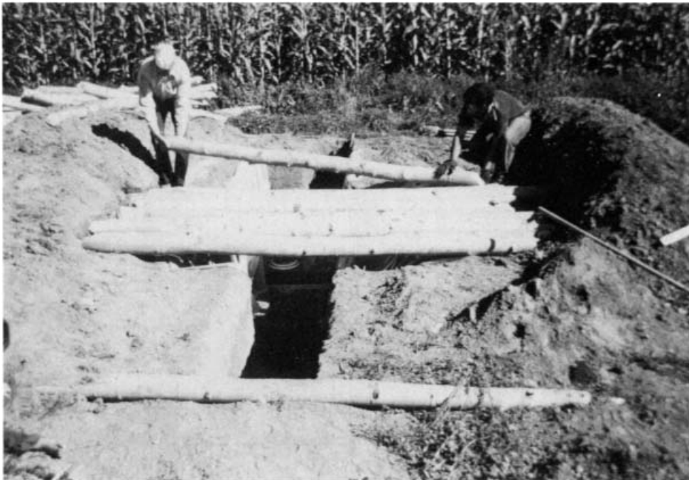
Fig. 5.1. Placing 9-foot poles for the roof of a Pole-Covered Trench Shelter.
